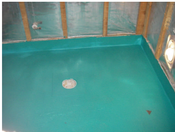
Saunan lattia on vedeneristetty.
